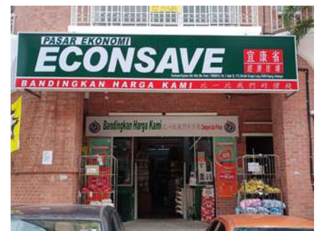
Six Eonsave sites in Malaysia achieve on average 20% energy savings September 2021 - March 2022.
