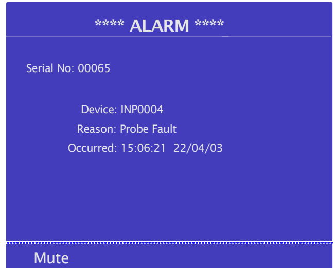
Typical alarm screen when not using PIN's to accept
